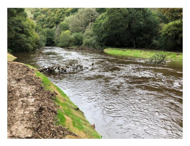
The work involved the removal of the concrete weir, sheet piling and gabion baskets, with approximately 60-65m of block stone removed along both banks.
